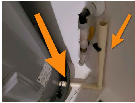
Drain to water heater pan not properly plumbed.
