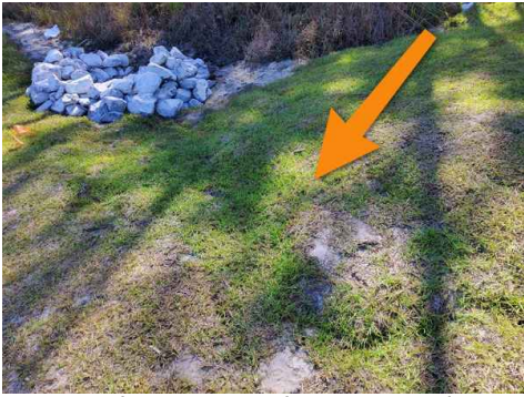
Erosion due to poor drainage. Sod needs to be removed and fill placed to correct erosion. Then sod should be replaced.
